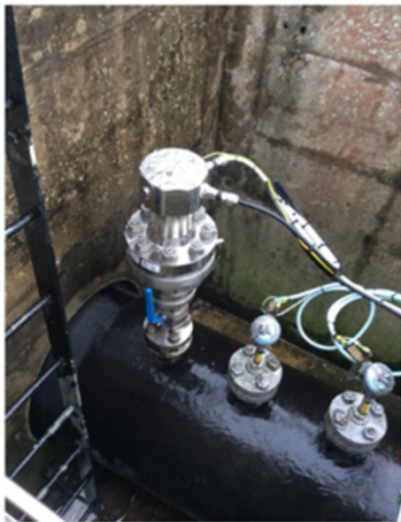
LineVu mounted on a pipeline and the view from the camera showing the pipe floor with dry gas
