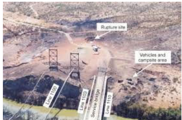
Figure 15b - Rupture site showing crater and bridge supports.
