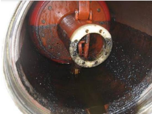
Figure 12. UK NTS routine pigging found ~ 100 litres, mainly TEG
