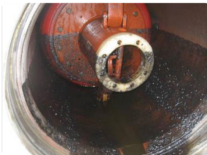
Figure 1. Result of pigging a “dry” network
